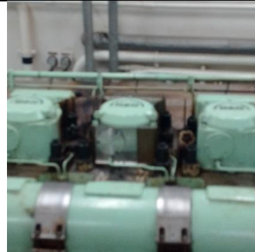
New installed No.7 cylinder cover
